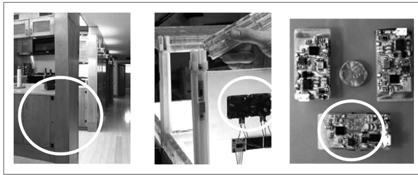
Figure 5 : Examples of sensors installed throughout the home
