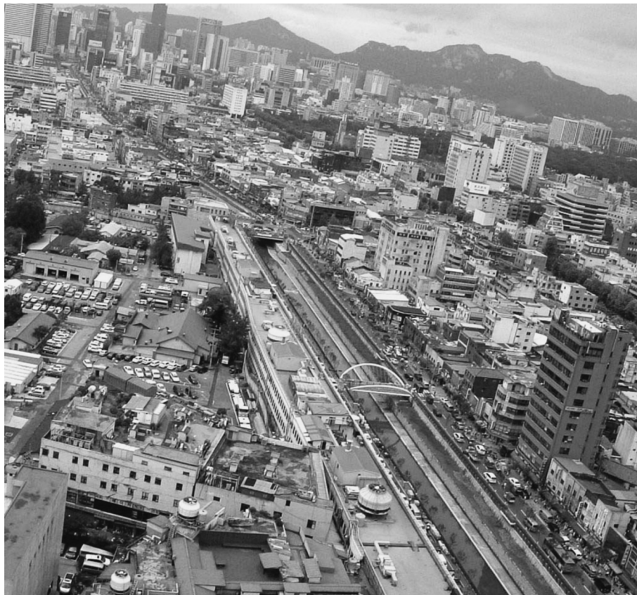
Figure 11 : Westward view from the rooftop of a building adjacent to the Cheonggyecheon near the Tondemun (August 2005) (see the color photo on the front cover)
