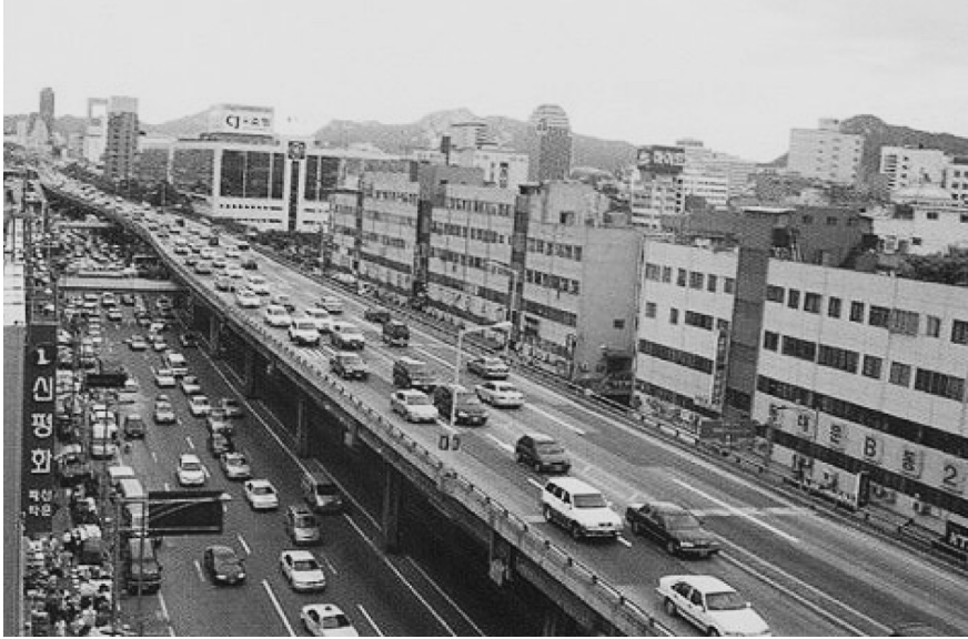
Figure 10 : Before restoration (the Tondemun district in June 2003)
