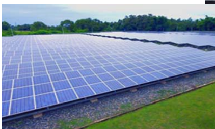
Rapid Deployment of 200 MW Solar PV Systems
