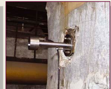
Photoelectronic torch sensors and oxygen gasanalyzer at the heat power unit
