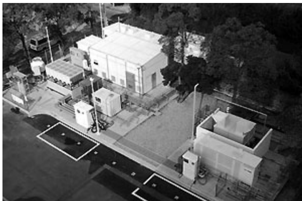
Figure 5: Hydrogen supply station (on-site hydrogen production type) based on the water electrolysis method [14]
